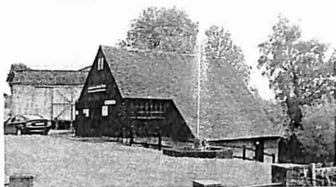
Coultershaw Beam Pump with fountain which is driven by the beam pump.
