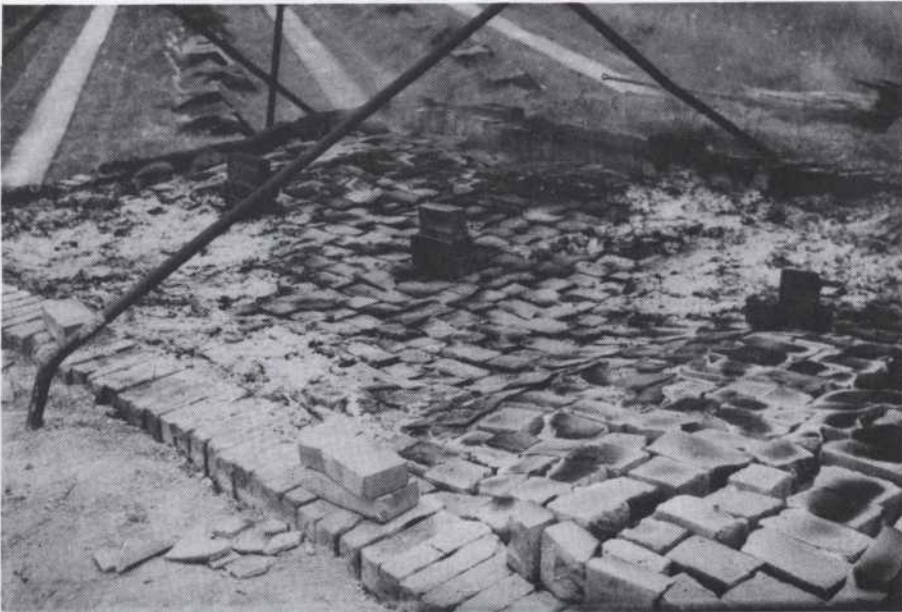
PLATE VI The Kiln top (Note the bricks for the levelling procedure and the nine tiles on the left.)
