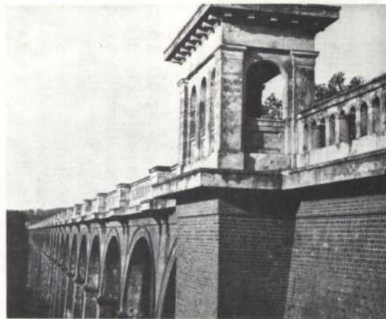
50 Ouse Viaduct, near Balcombe
