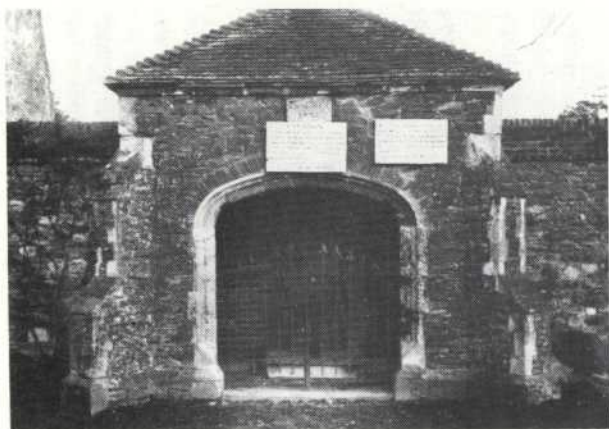
150 Town Well and Well-House, Winchelsea
