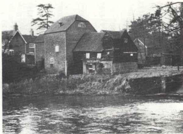
118 Terwick Mills, near Trotton
