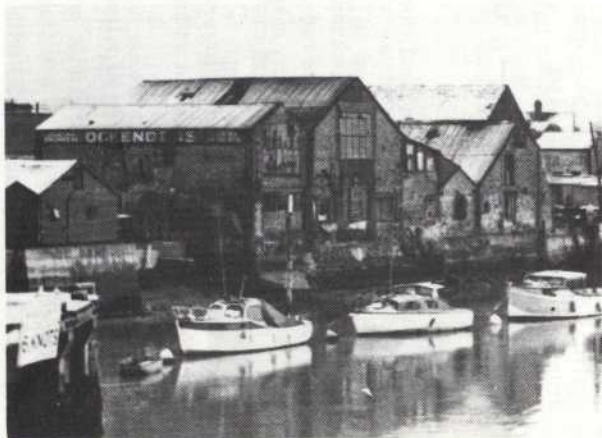
75 Workshops in River Road, Littlehampton
