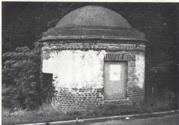
22 Tollhouse at Ashcombe
