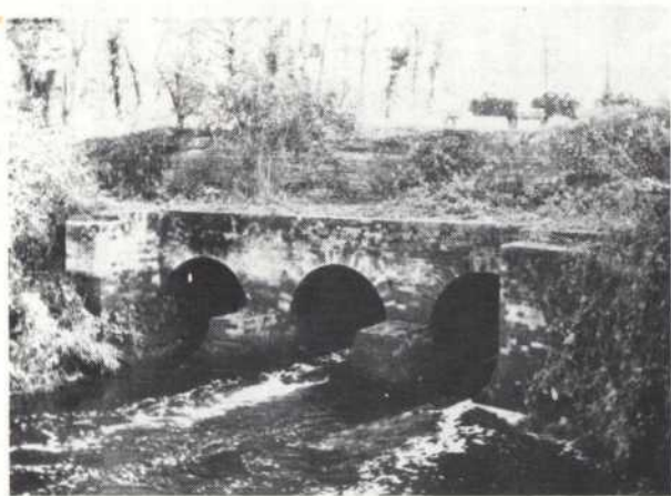
43 Orfold Aqueduct, Arun Navigation
