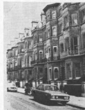
Fig. 6 Nos. 18 to 26 First Avenue
