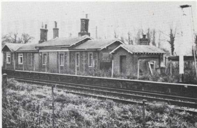
PLATE 2: Woodgate: station for Bognor from 1846 to 1864.
