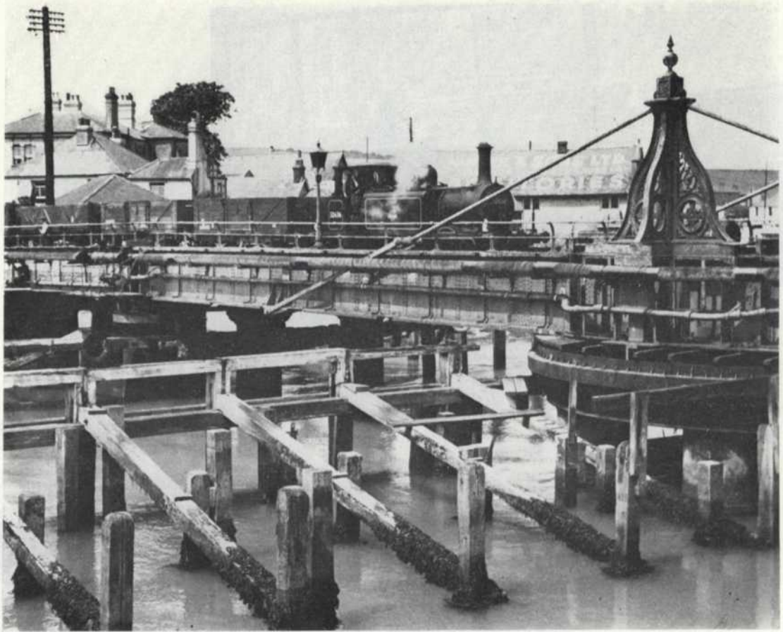
Plate X Freight train crossing the bridge (R. C. Riley).
