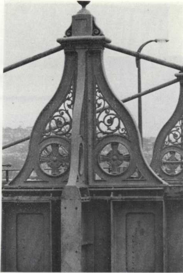
Plate IV Central iron structure for tie rods.
