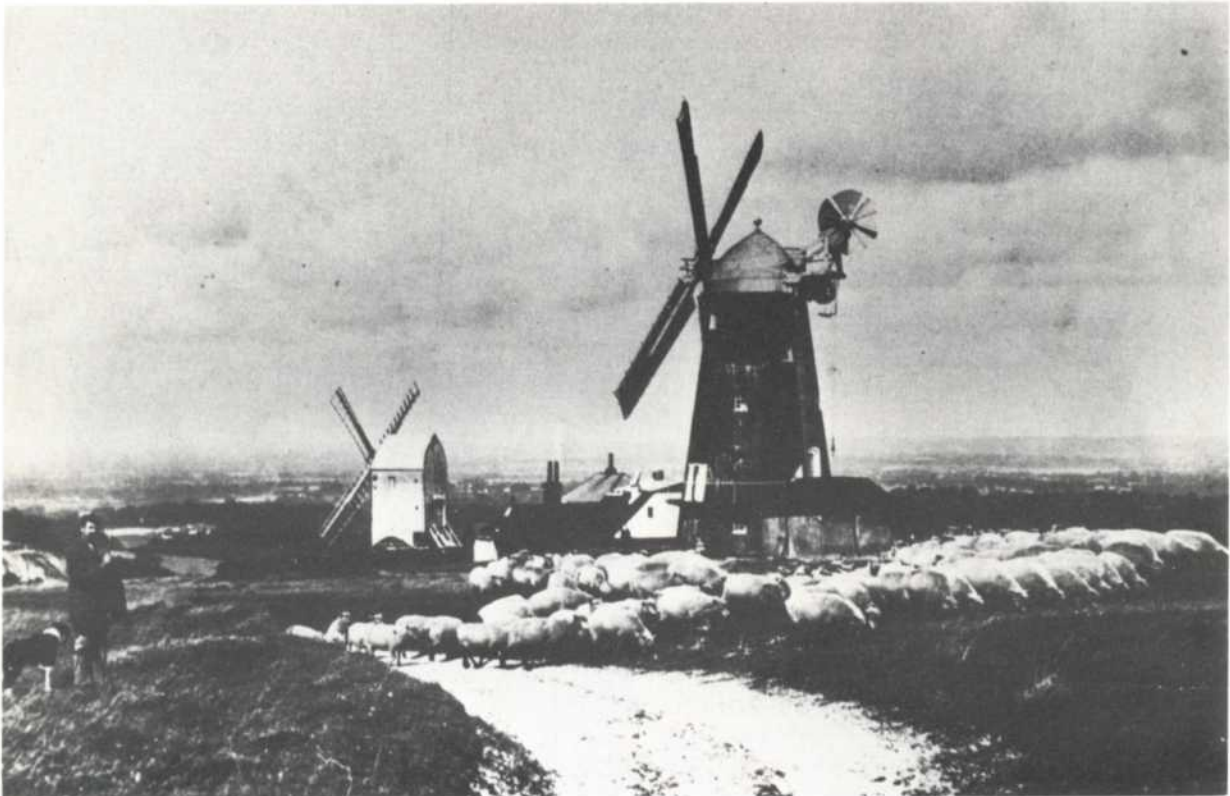
Jack and Jill in 1905. The round house of Duncton Mill next to Jack's tower.
