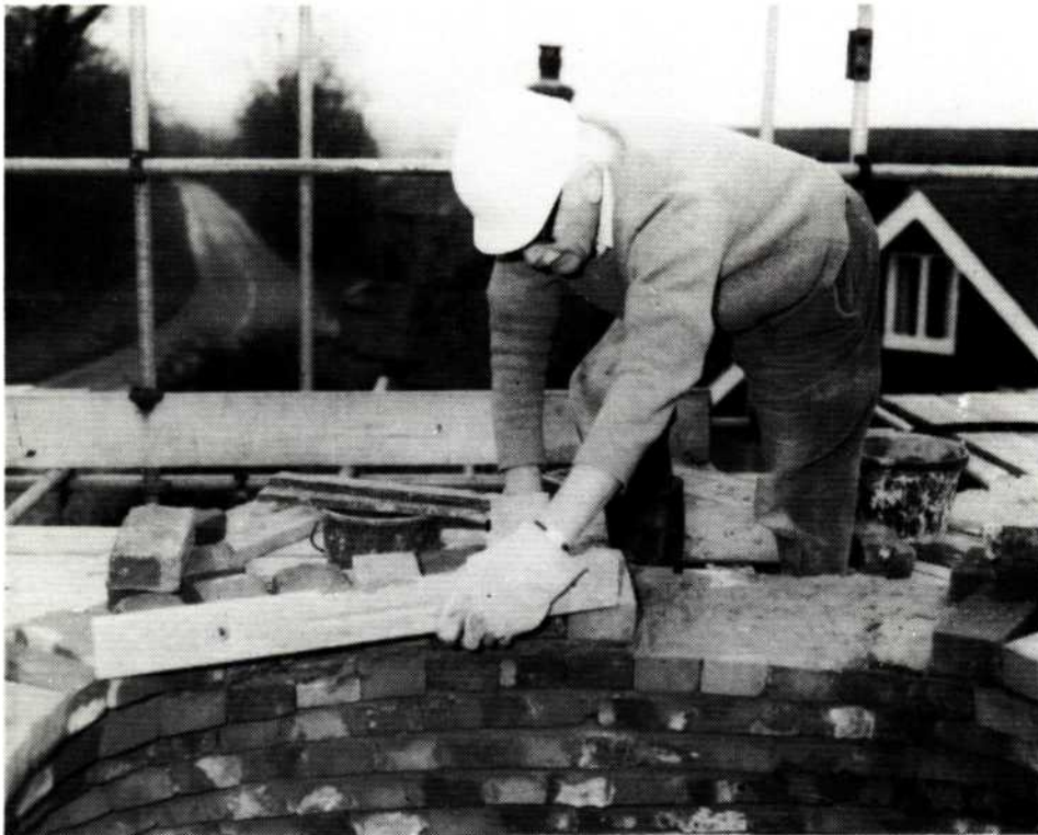
Fig. 6 Checking Levels
