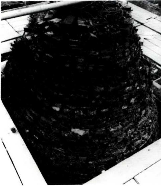
Fig.5 Top of Kiln Before Restoration
