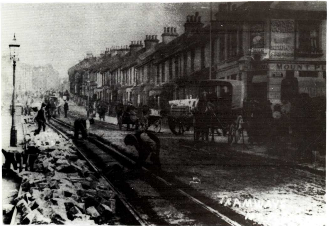
Fig. 1 Track Laying in Mount Pleasant Road (Courtesy of Hastings Museum)
