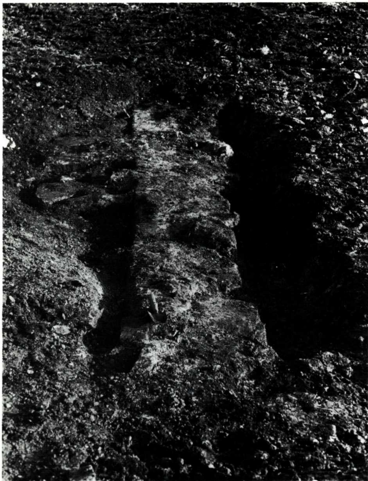
Fig. 3 The Sandstone Wall at Westfield Forge.
