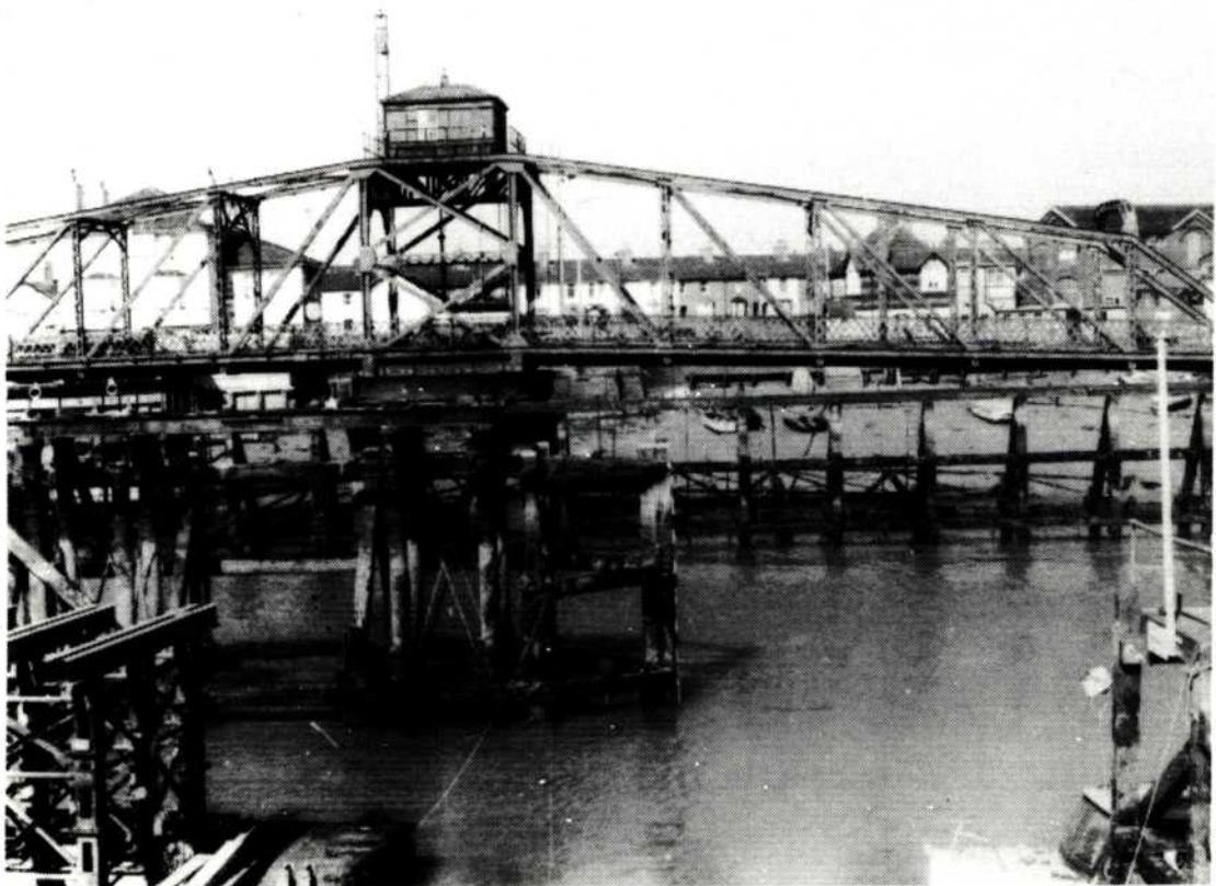
Fig. 1 East (Movable) Span of Bridge
