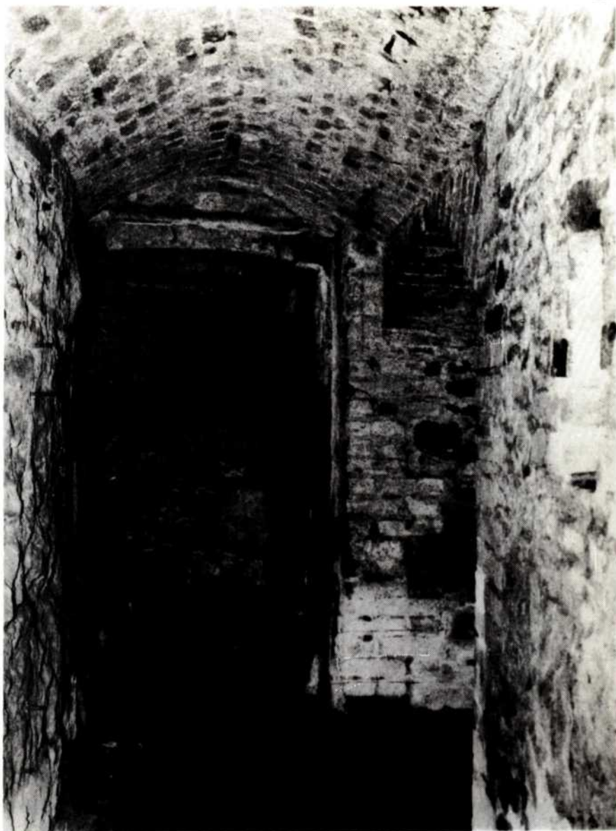
Fig. 1. Entrance Passage to Ice-House.
