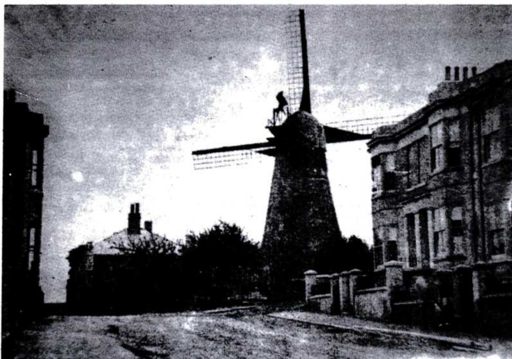
A photograph taken about 1853 shows that Hodson's Mill was still complete with four canvas cloth sails and fan-tail. Houses had been built close by, and these must have affected working on calm days.
