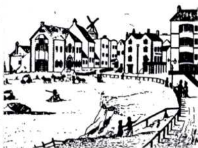
West Street Mill viewed from Old Steine From a View of Brighthelmstone by J Watts, 1785
