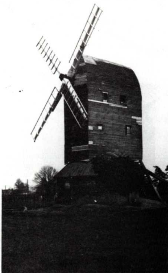
Fig.6 After the new sails had been fitted in 1938. It is a shame that the ivy wasn't removed as well.
