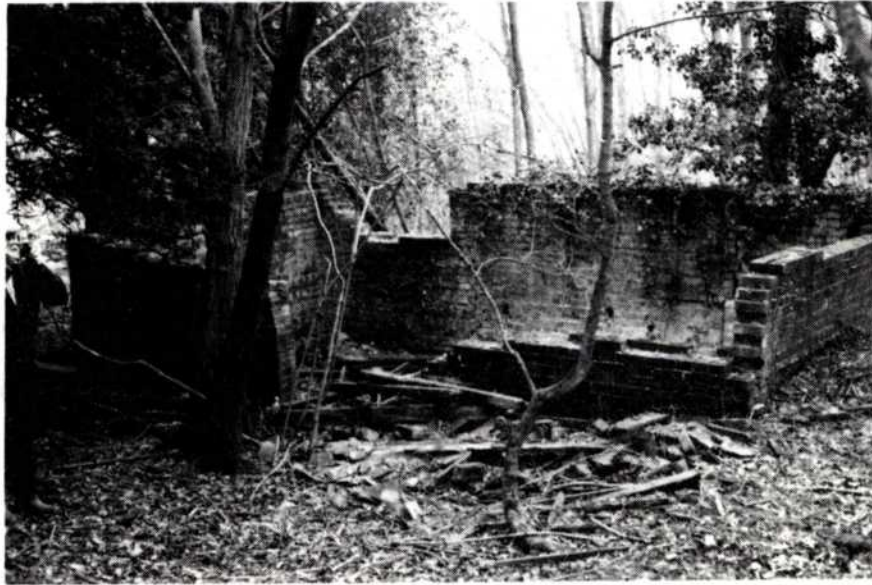
Fig.4 Bignor Park Pumphouse as found 1985.
