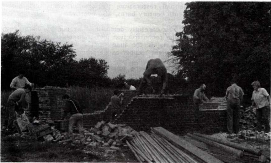
Fig.12 Volunteers hard at work demolishing the roundhouse.
