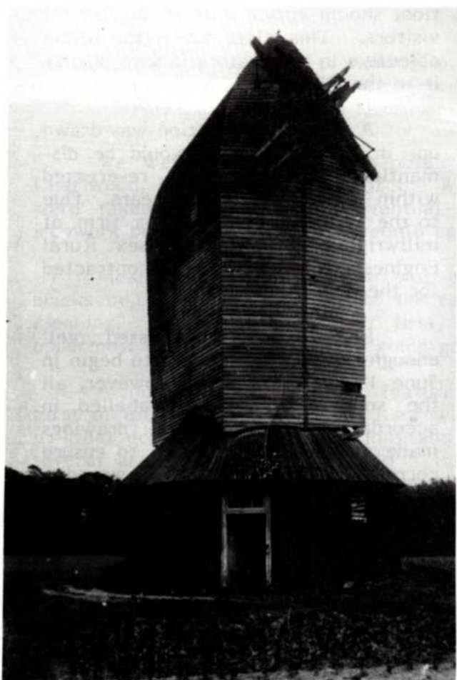
Fig.5 Circa 1923, note the corbelling in the roundhouse brickwork.
