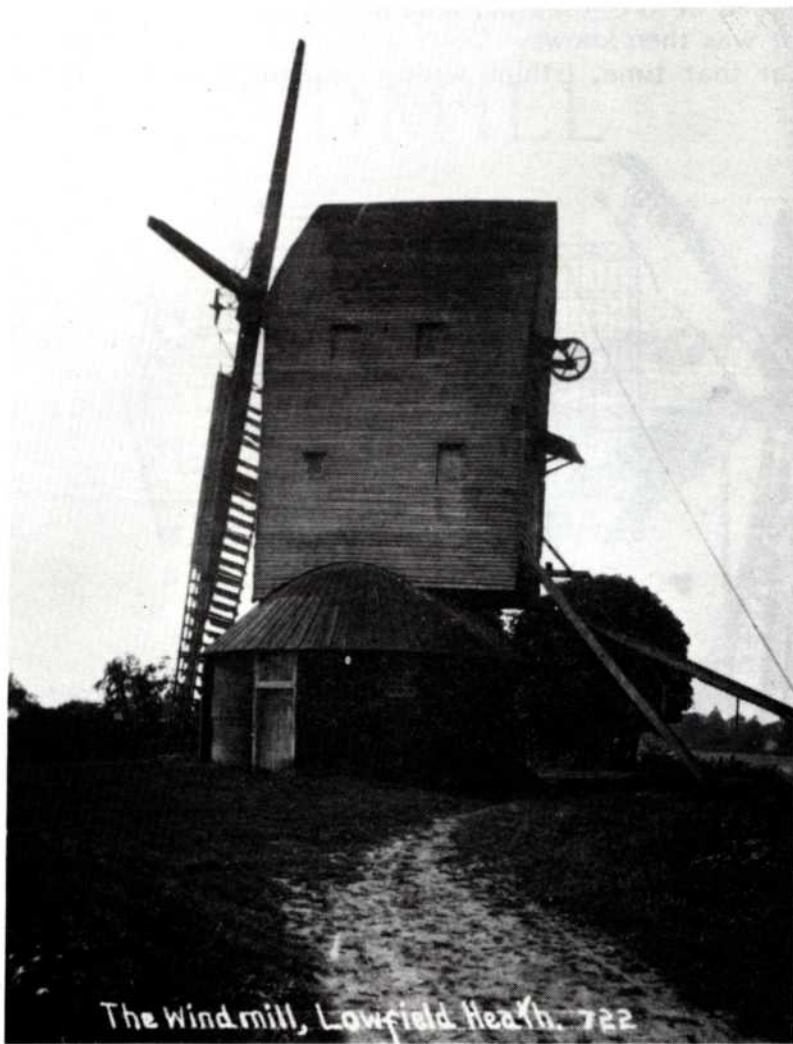
Fig.2 Circa 1900. Note the striking chain weight sitting on a small platform below the chain.
