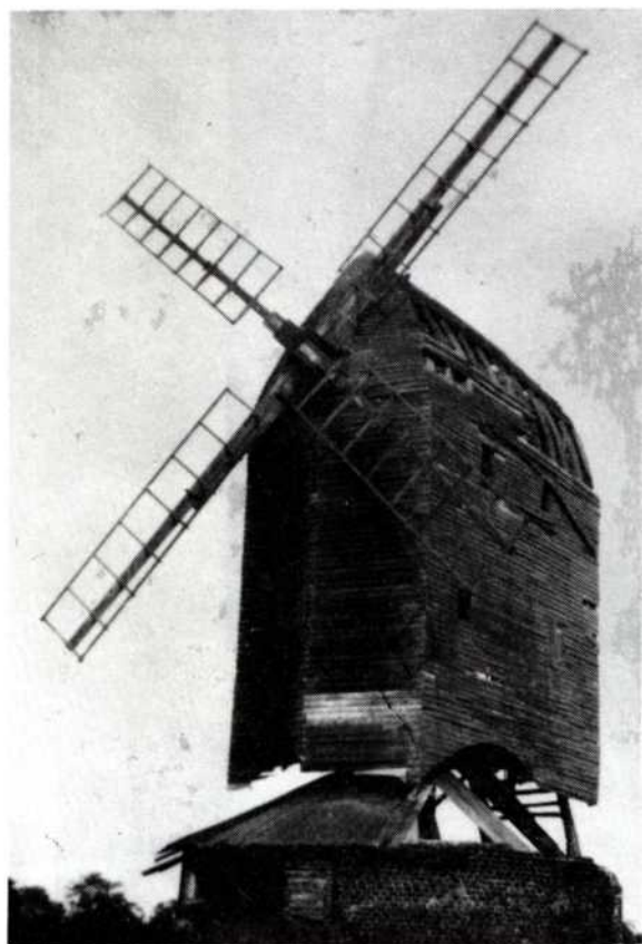
Fig.7 Circa 1950 with the roof obviously starting to rot.
