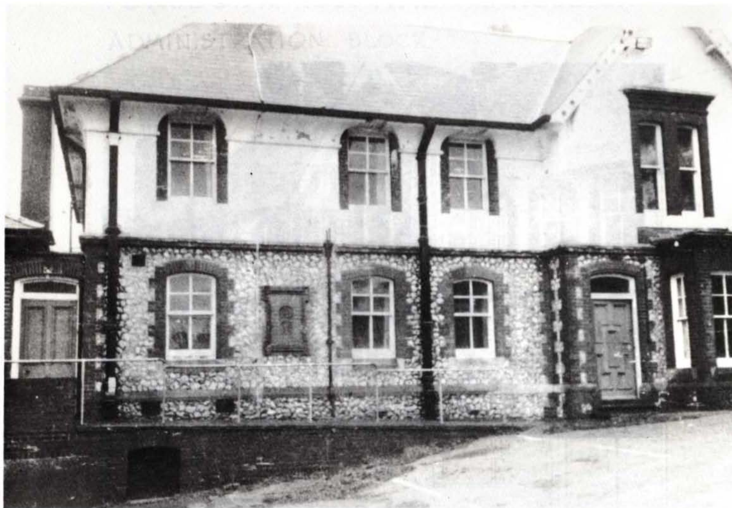
Fig.4. North-west elevation of the administration block
