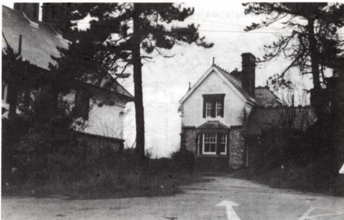
Fig.7 The lodge (centre) with part of the administration block (left)
