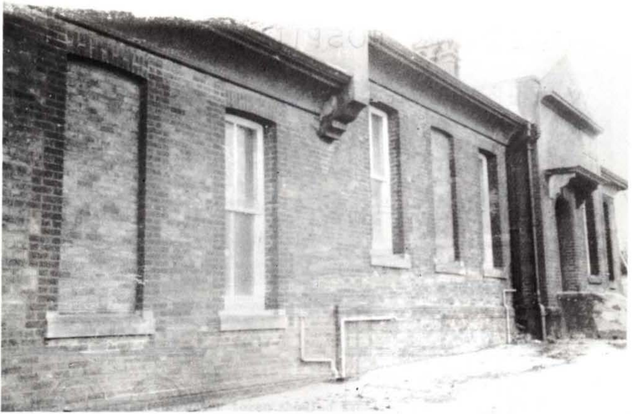
Fig.9 North-east elevation of ward block EF of 1912
