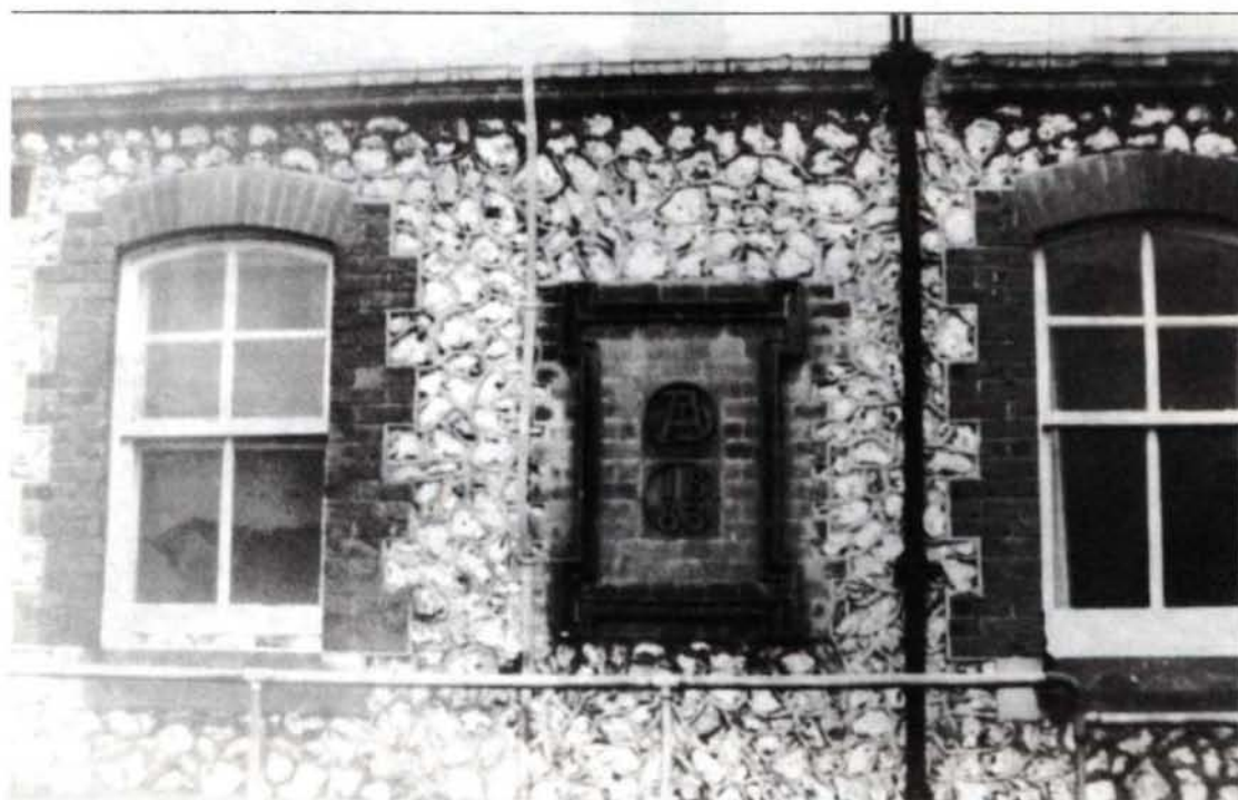
Fig.5. Plaque with date "AD1883" on north-west elevation of the administration block
