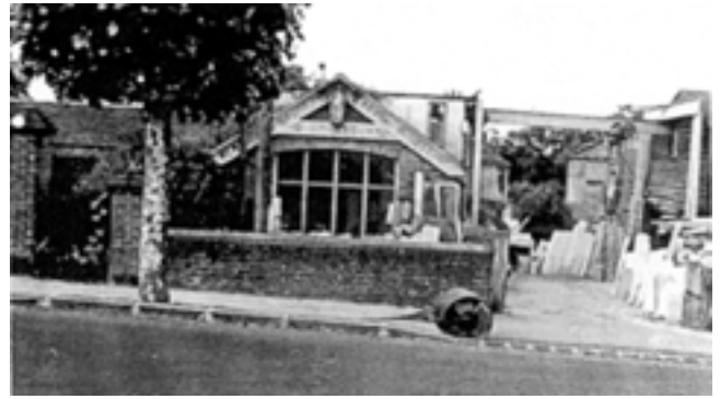
Fig.5 Stonemasons' Yard on the western side of London Road
