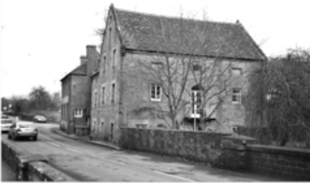
Fig. 4 The west face of the main mill buildings today, looking north. In the apex of the gable is set a date-stone which is now illegible. The 1806 mill cottage lies beyond. (Author)
