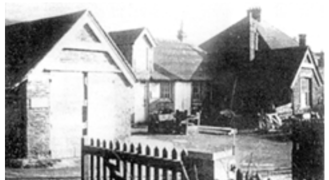
Fig.6 Blacksmiths and paint stores on the eastern side of London Road
