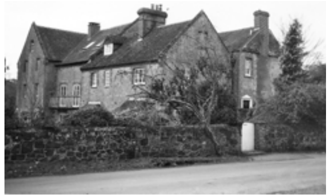
Fig.7 The mill buildings today, viewed from the north east, with the lane leading to Cowdray House in the foreground. The part of the building to the right with the chimney in its gable is the 1806 cottage now called Mill Cottage which, to its south, is abutted by the main part of the 1840 buildings now known as North Mill. To the east of the 1806 cottage is more of the 1840 rebuild now called North Mill House. The mill race passes below the two balconied casement windows. (Author)
