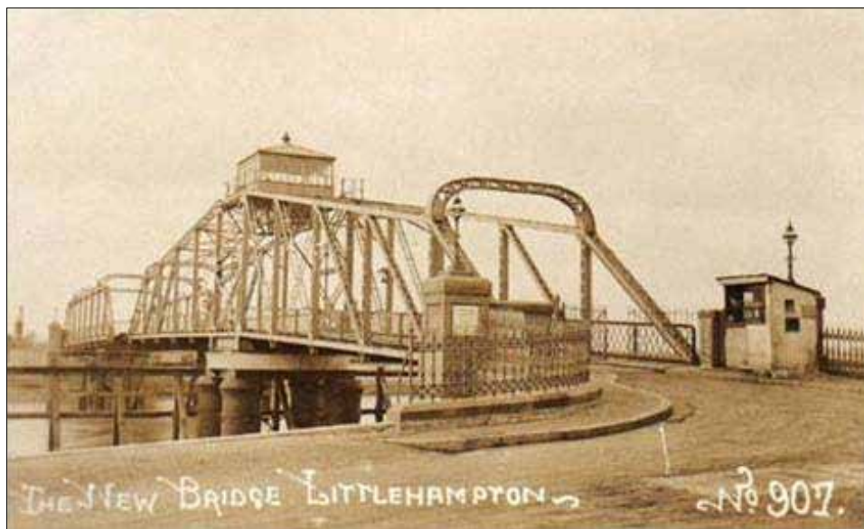
1908 view with original toll booth
