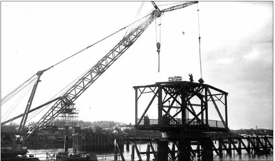
Littlehampton swing bridge dismantling - last days 1980, note floating crane
