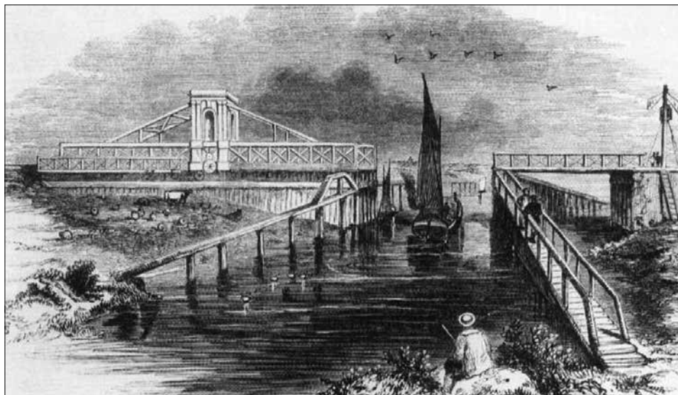
1846 LBSCR wooden rail bridge at Ford
