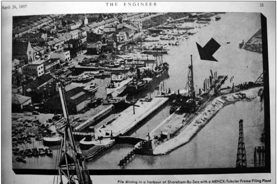
Pile Driving at Locks at Shoreham Harbour 1957
