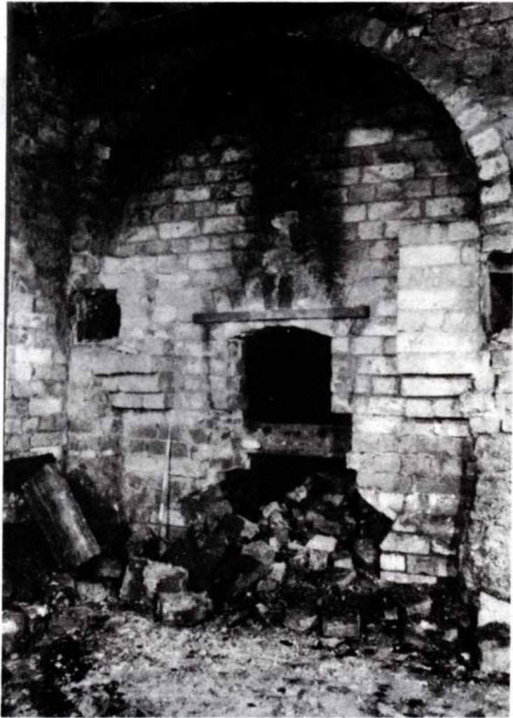
Fig 12. Front of the north fire box at level 1 (Nick Catford)
