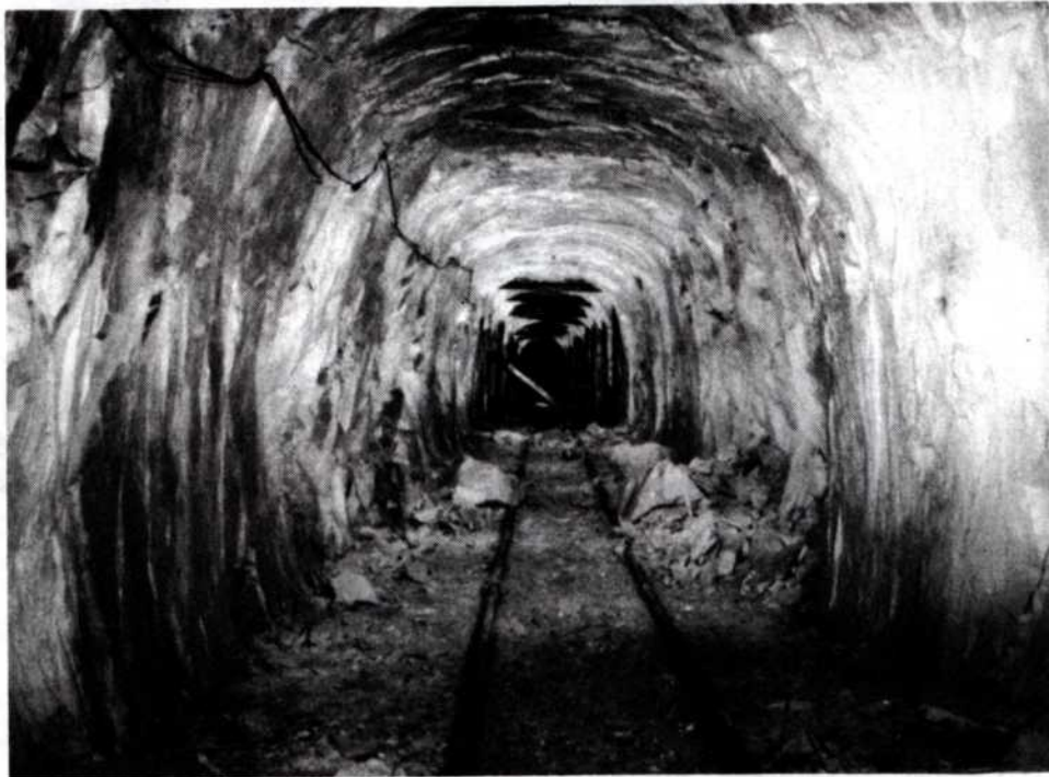
Fig 15. Tunnel at level '0', looking west (Nick Catford)
