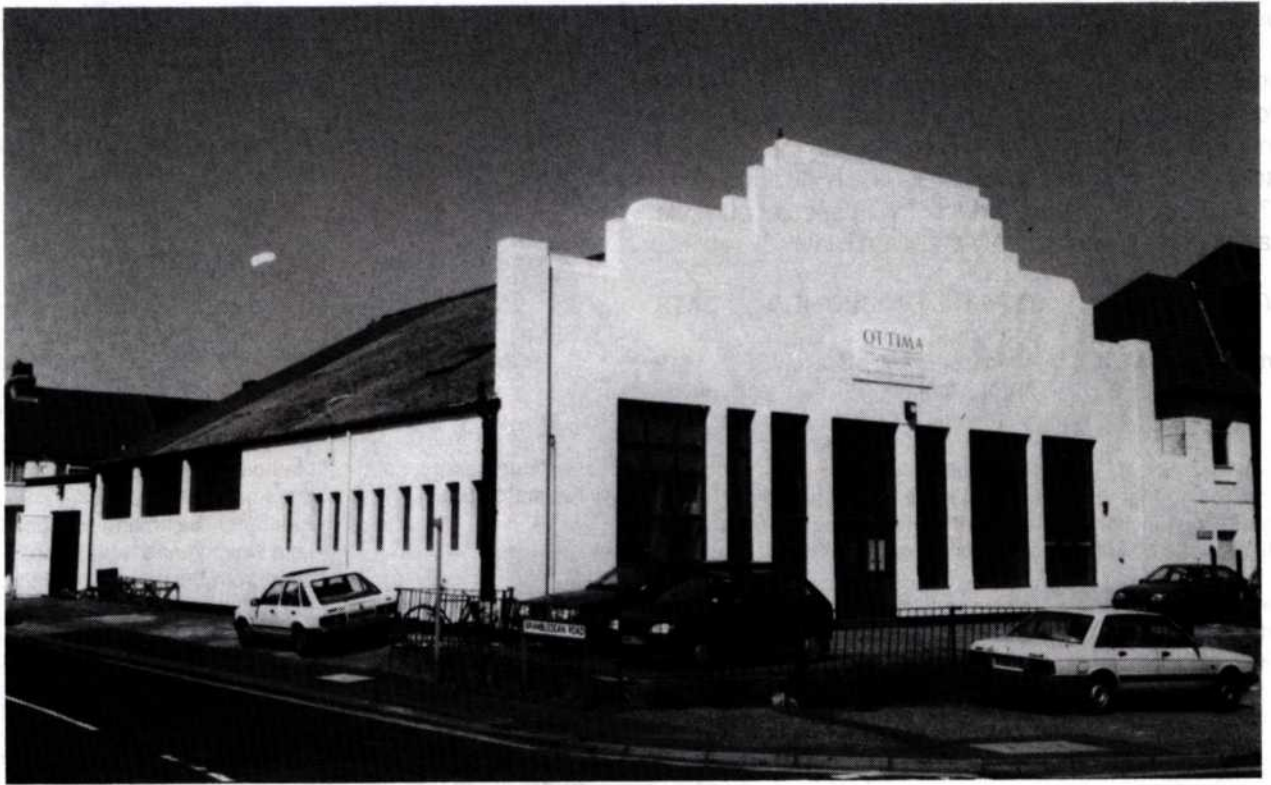
Fig. 17 Garage building on the corner of Brambledean Road, Portslade used by E.H. Jones c.1949-55
