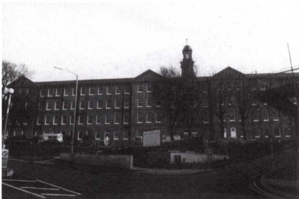
Fig. 4 Brighton General Hospital Arundel Building "A" Block, built 1866
