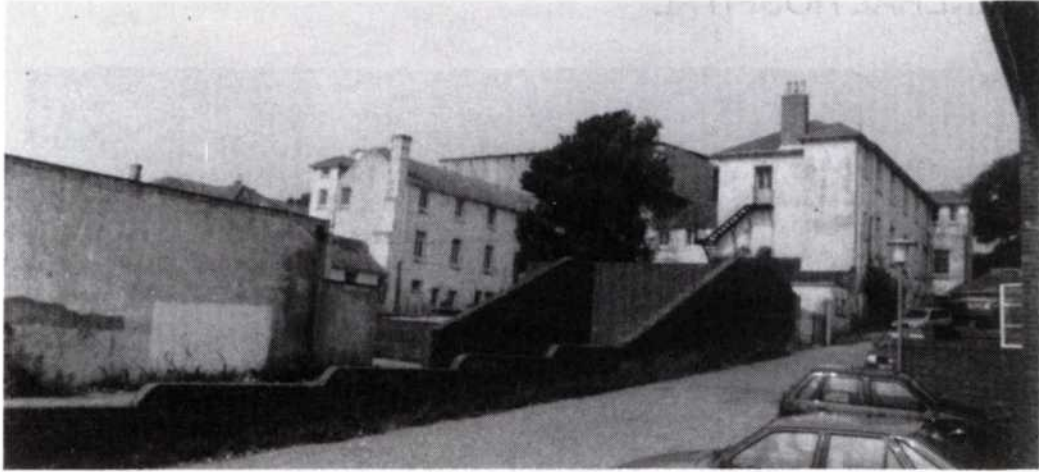
Fig. 2 Rear (South East) Elevation, Warren Farm Industrial School
