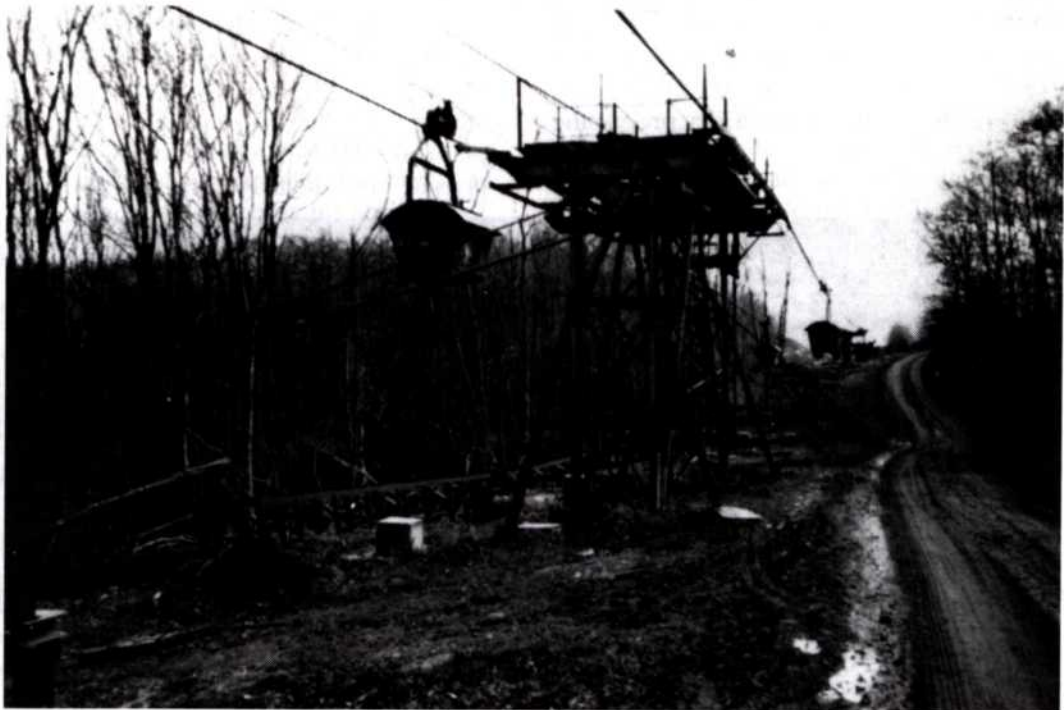
Fig. 6 Steel fabricated tower on the Brightling to Mountfield cableway, showing the typical terrain traversed. Photograph taken 1988 just before its replacement by a continuous conveyor belt costing £6 million. (W.R. Crawshaw)
