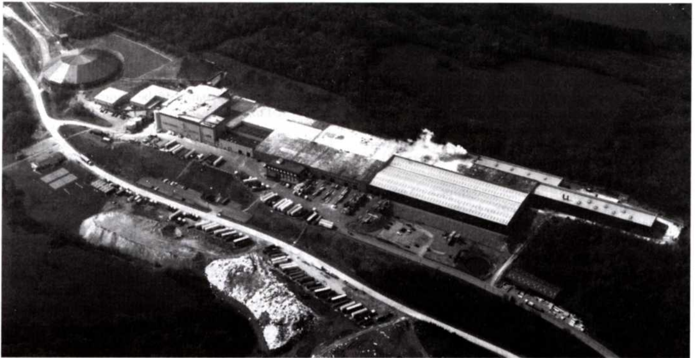
Fig. 3 Aerial View of Mountfield Gypsum Works from recent photograph supplied by British Gypsum Ltd. Head Office at Loughborough
