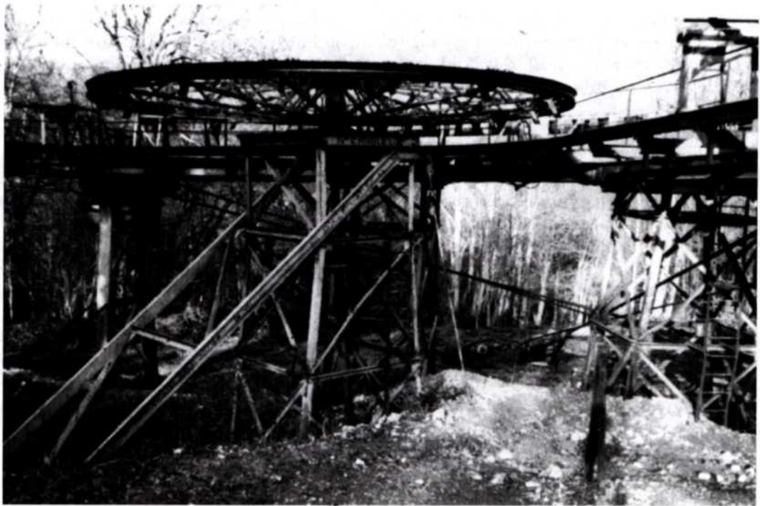
Fig. 5 Steel fabricated change of direction station on the Brightling to Mountfield cableway, taken 1988. (W.R. Crawshaw)
