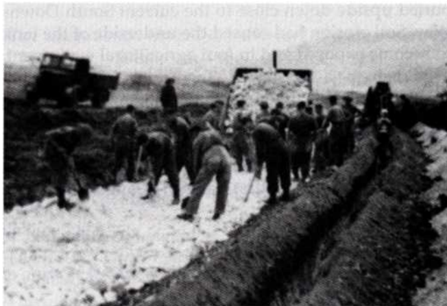
Royal Engineers laying a labour intensive WWII tank road on the remote South Downs.
