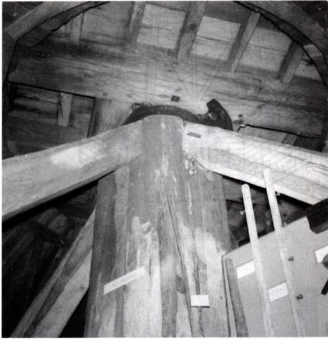
Fig. 10 Argos Hill Mill – centre post entering body of mill
