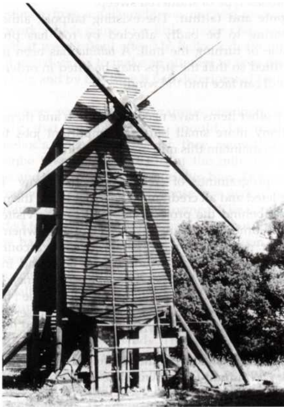
Fig. 60 Nutley Mill – showing the two brick piers (Brian Austen)
