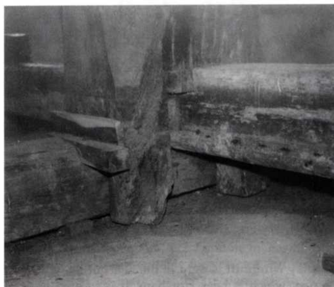
Fig. 32 Base of the High Salvington centre post
