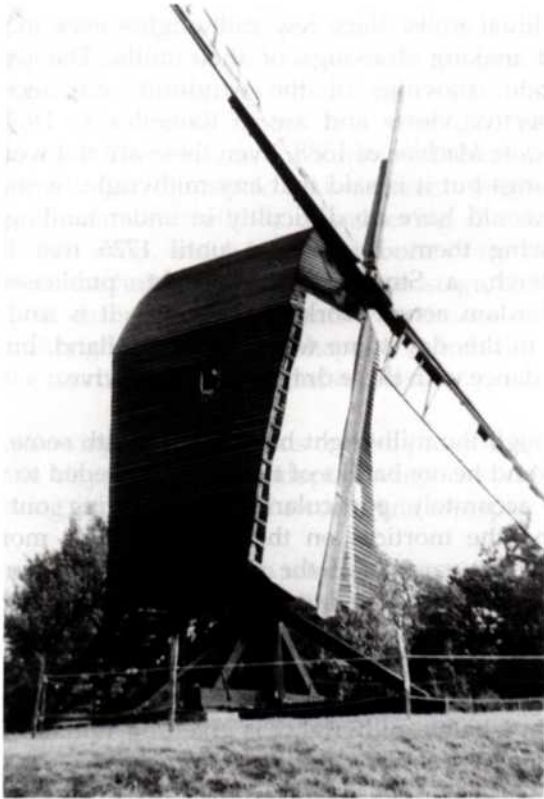
Fig. 15 Common and spring sweeps of Nutley Windmill (H. James)
