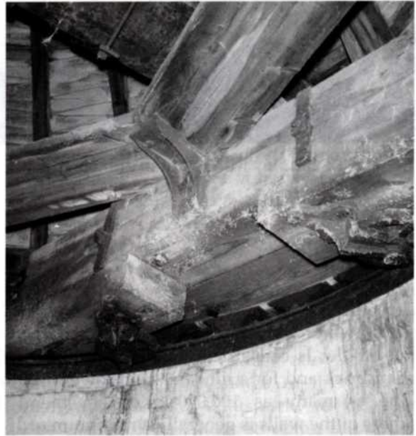
Fig. 11 Curb and centering wheels
