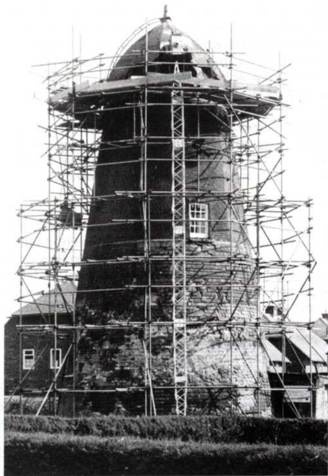
Fig. 65 Polegate – Renovations in progress (Lawrence Stevens)
