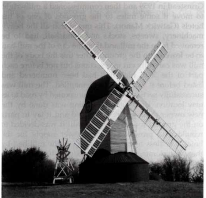
Fig. 23 Argos Hill with new stock and sweeps
