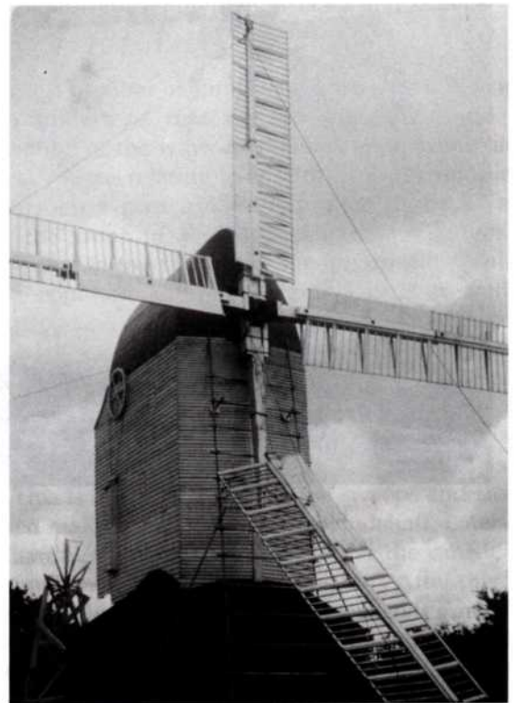
Fig. 19 Argos Hill Mill – first sweep being lowered
