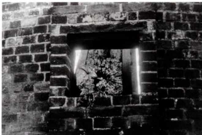
Fig. 71 Cross tree protruding through the roundhouse wall, Lowfield Heath
