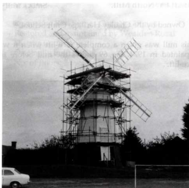
Fig. 70 Chailey – extent of the scaffolding necessary when painting a windmill
