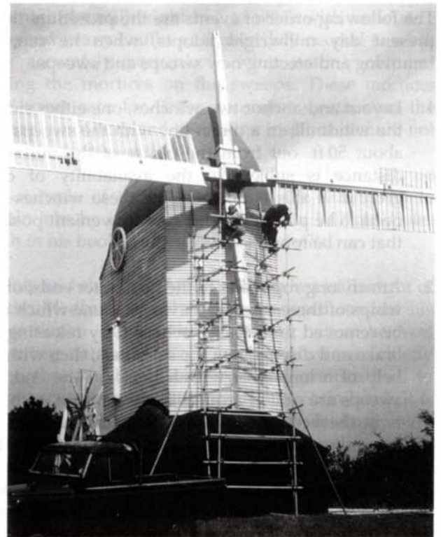
Fig. 21 Extra scaffolding being erected
