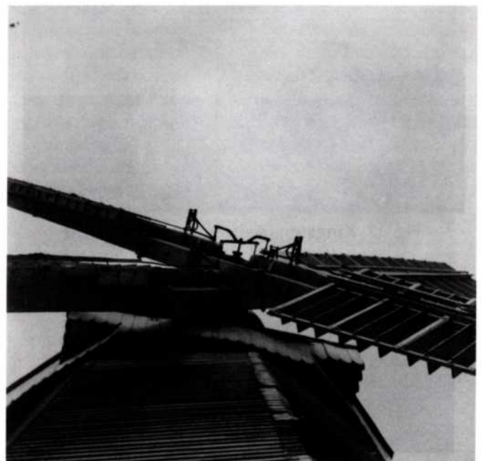
Fig. 16 Shipley Mill – patent sweeps
