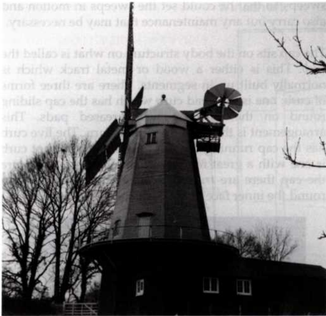
Fig. 12 Shipley Mill – fantail and staging
