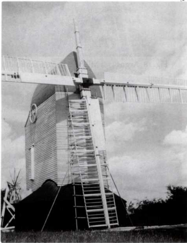
Fig. 20 Argos Hill Mill – second sweep being removed
