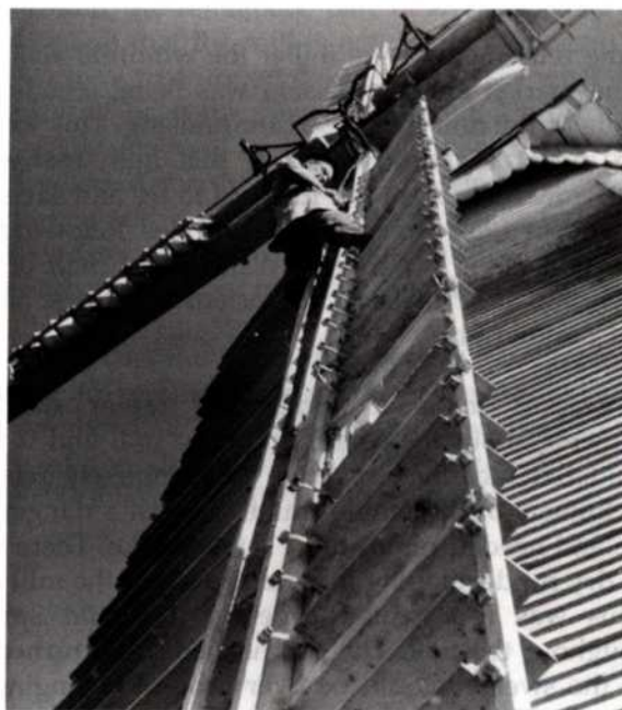
Fig. 63 Shipley – showing shutter linkage and a millwright working on the sweeps
