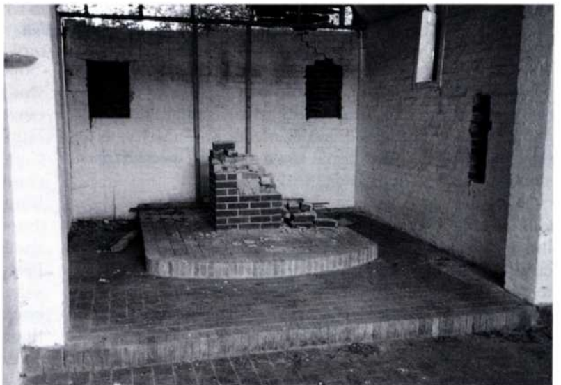
Fig. 5a and b Exterior and interior views of the redundant chapel.
