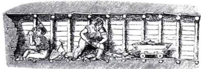
Fig. 7 Driving the headings. F.W. Simms, Practical Tunnelling .
