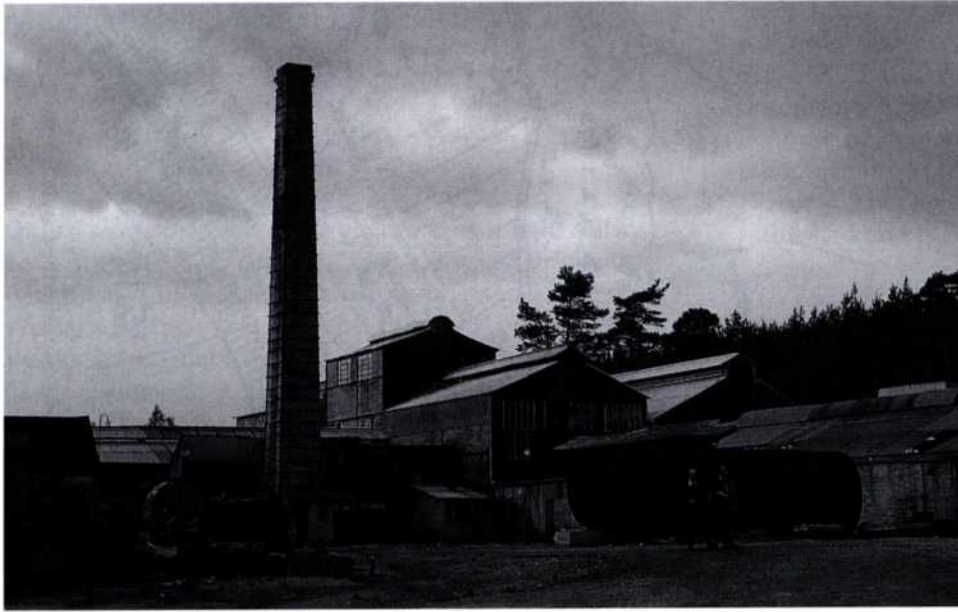
Fig. 2 General view of the Works showing the 85 ft. chimney stack erected c.1926. Photo: Chris Bryan
