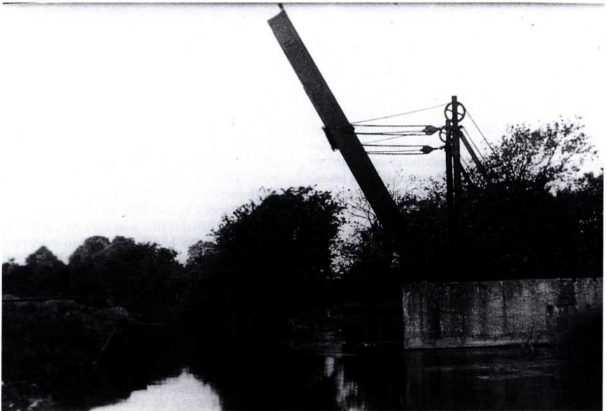
Fig. 4 The same view with the bridge raised (Chichester Museum)
