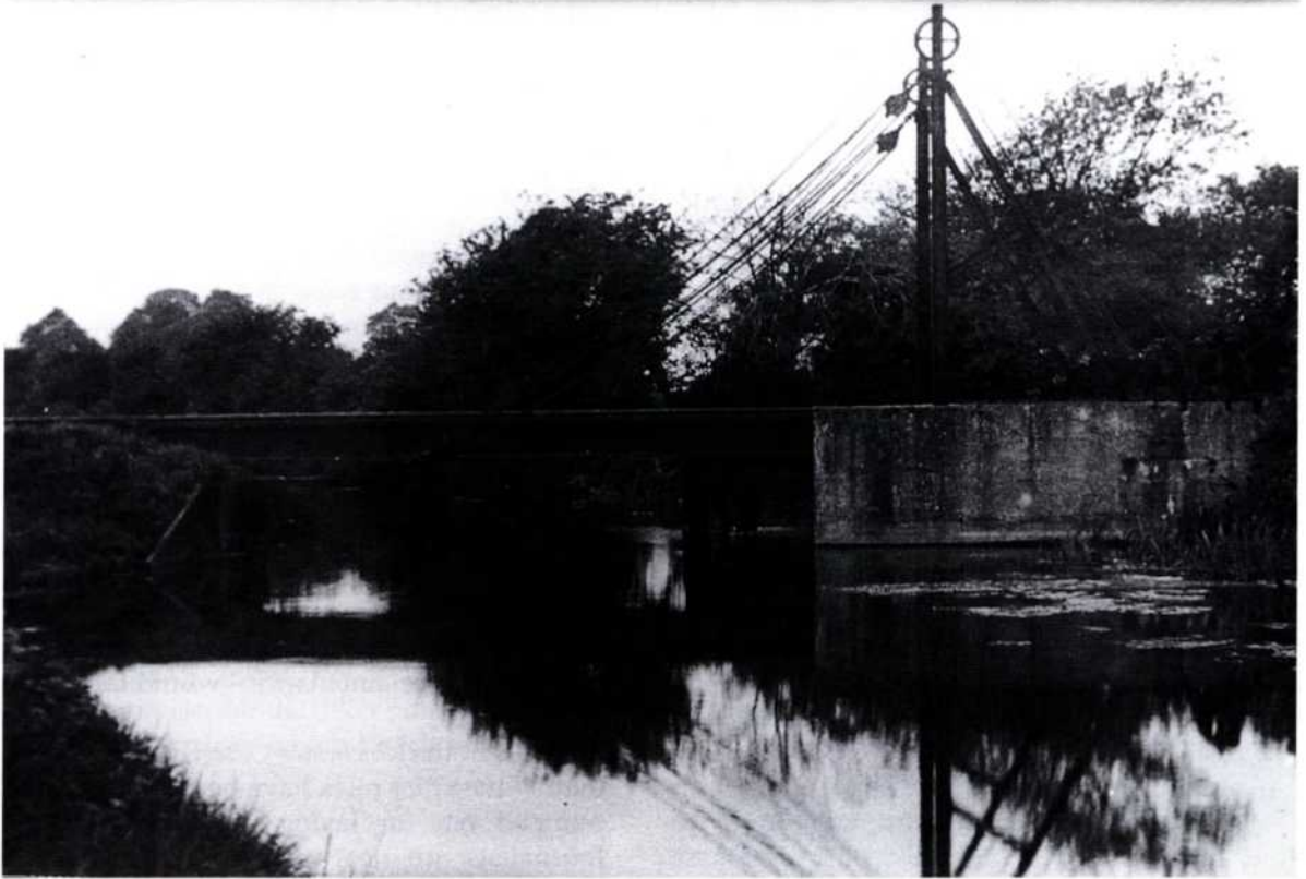
Fig. 3 A view of the bridge looking east, note the four falls of chain. (Chichester Museum)
