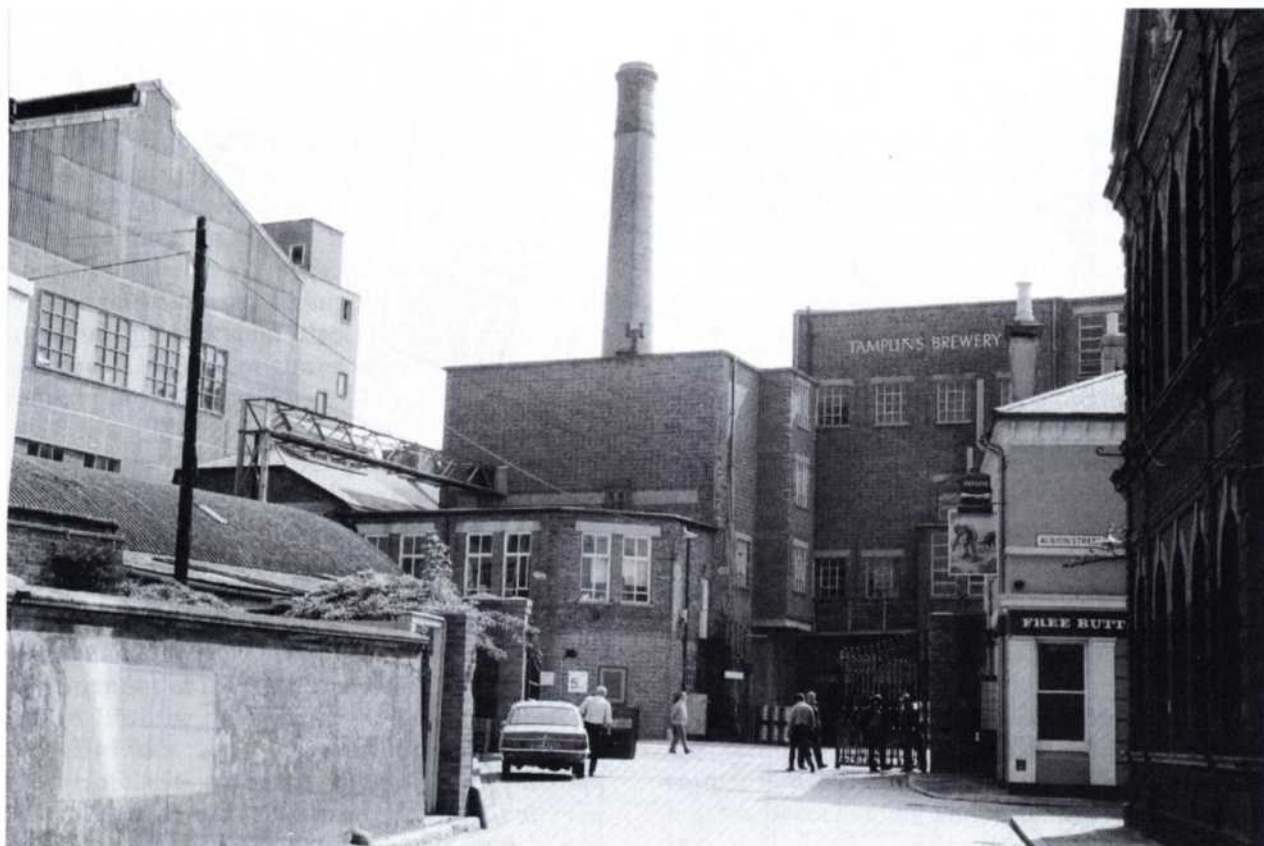
Fig. 1 Brewery Buildings from Phoenix Place, August 1976
