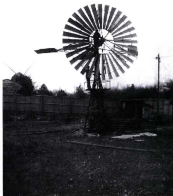
Fig. 2 Wind generator with dynamo shed at base, and standby engine shed to the right. A distribution pole with wire and insulators stands nearby. The main shed, divided into store, battery room and switchroom can just be seen in the left background.
