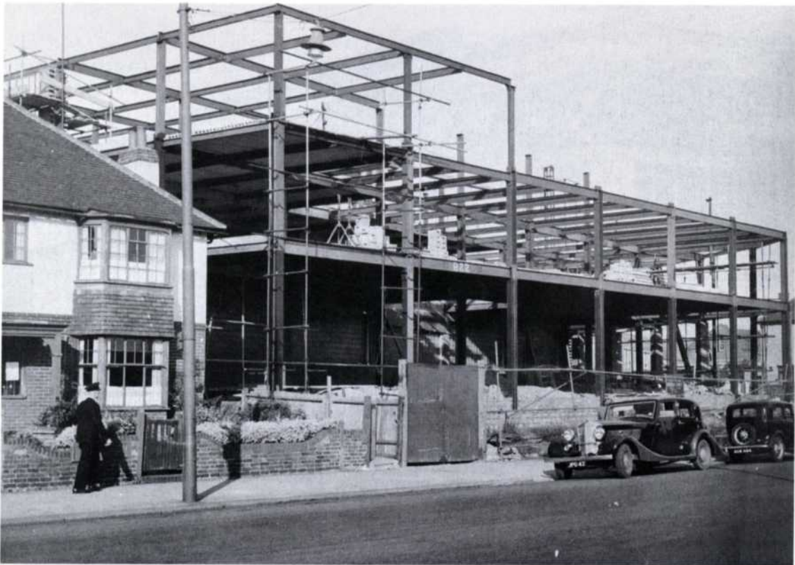
Fig. 8 Steel construction work proceeding on the Portland Road site
