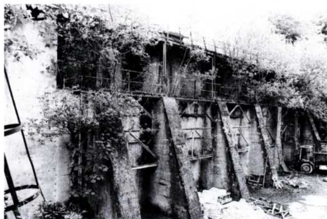
Fig. 2 Cocking Lime Works. General view of South Battery of kilns.
