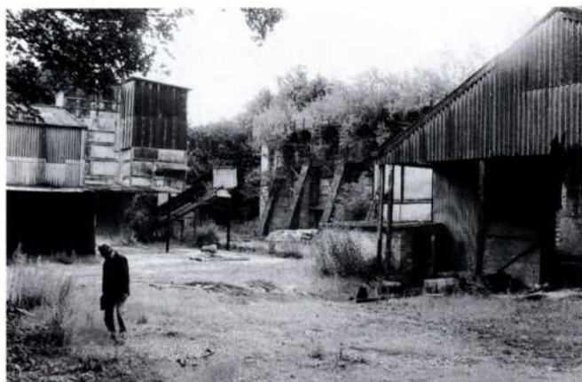
Fig. 1 Cocking Lime Works. General view of lower site.
