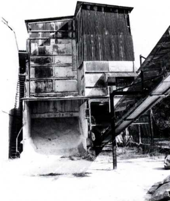
Fig. 5 Cocking Lime Works. Screening Plant
