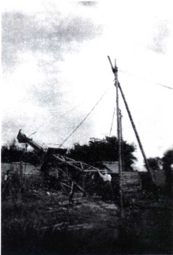
Fig. 3 Generator being taken down before removal to rear of 16 Heather Lane December 1924.
