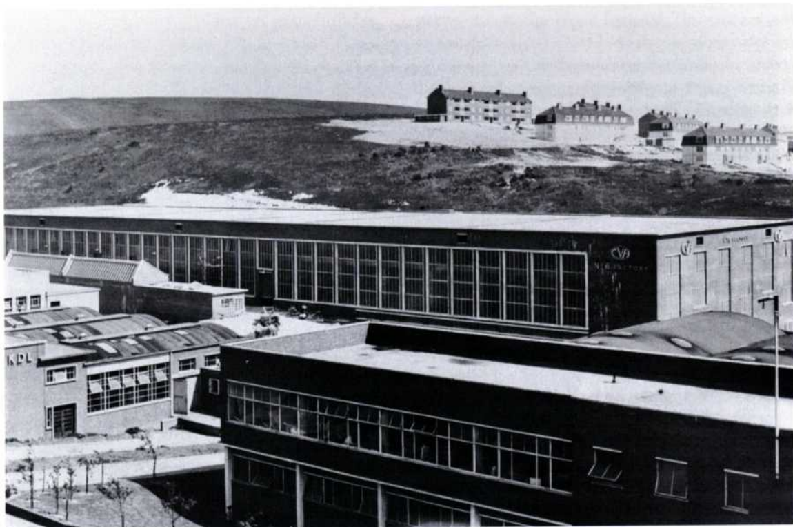
Fig. 17 CVA No. 6 factory after completion
