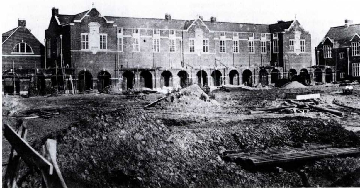
Fig. 2 Cloisters and classrooms under construction.
