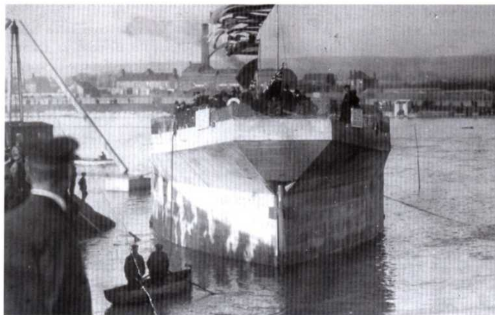
Fig. 4 Stern view of the barge Crestile being floated out of its basin 18 January 1919
