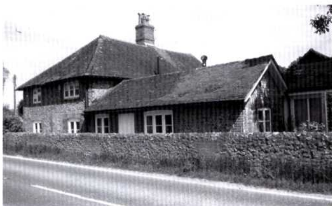
Fig. 7 Upwaltham tollhouse (John Blackwell)
