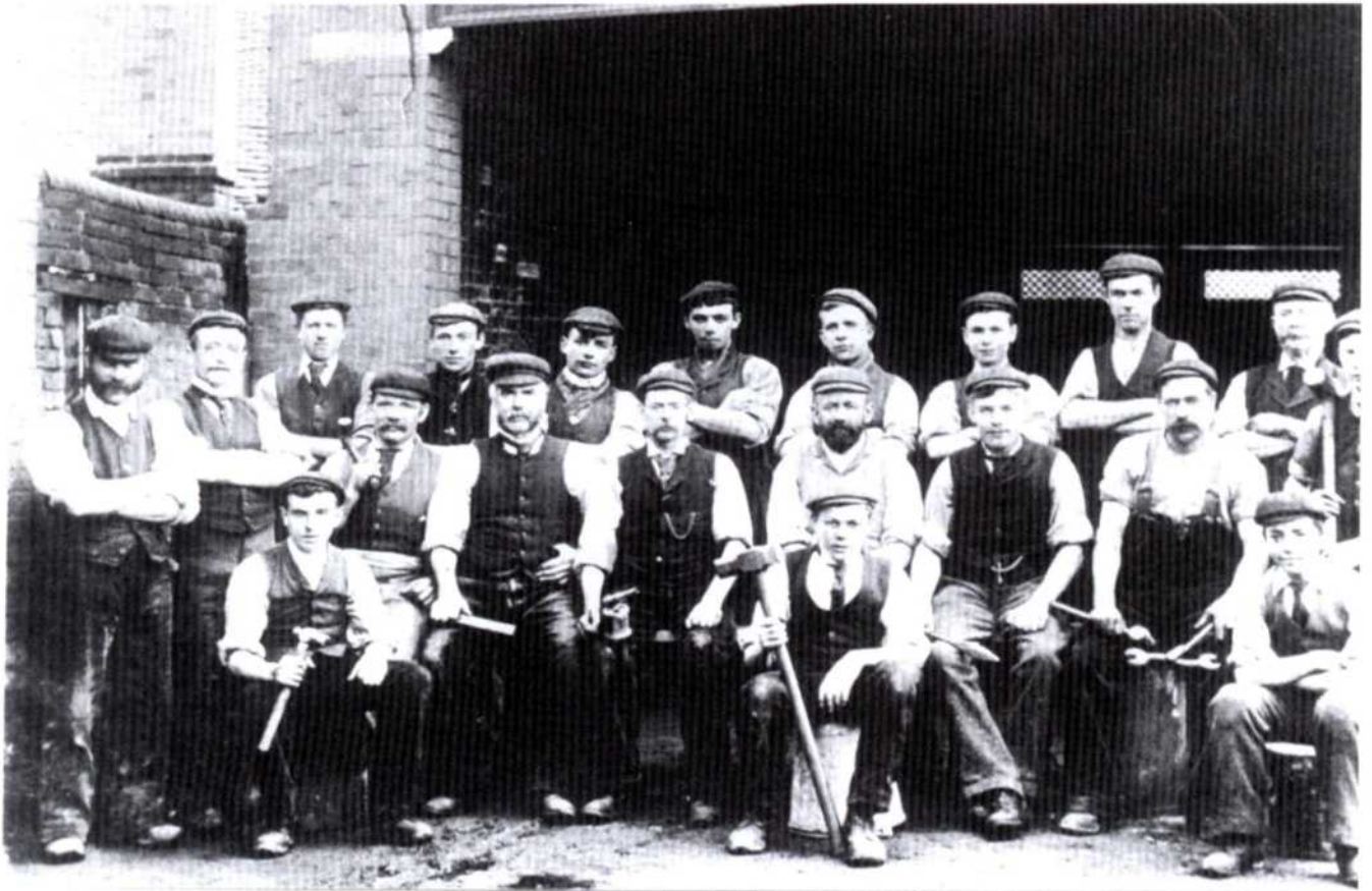
Fig. 13 The assembled workforce staff of Halsted & Sons. They are gathered with the main gates of the site as a backdrop; all are sporting waistcoats and most of them ties as well! Note the pier to the left supporting the cast-iron beam to the building which used to span the entrance – it is all that now remains of this scene. (Bernard Price collection)
