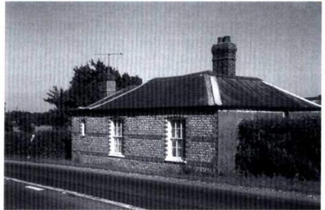
Fig. 8. Clay Lane, Storrington tollhouse
