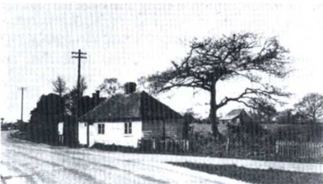
Fig. 5. Dial Post tollhouse prior to its demolition in 1937 (Weald and Downland Open Air Museum)
