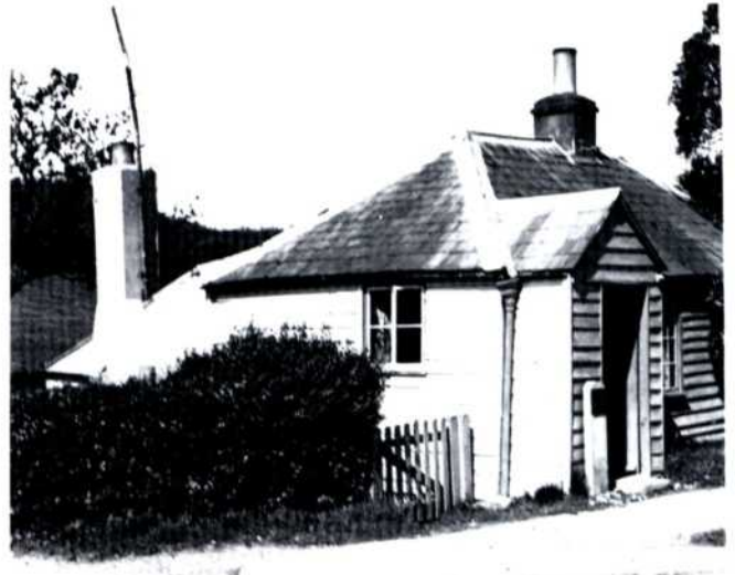
Fig. 4. Findon tollhouse photographed 15 May 1938
