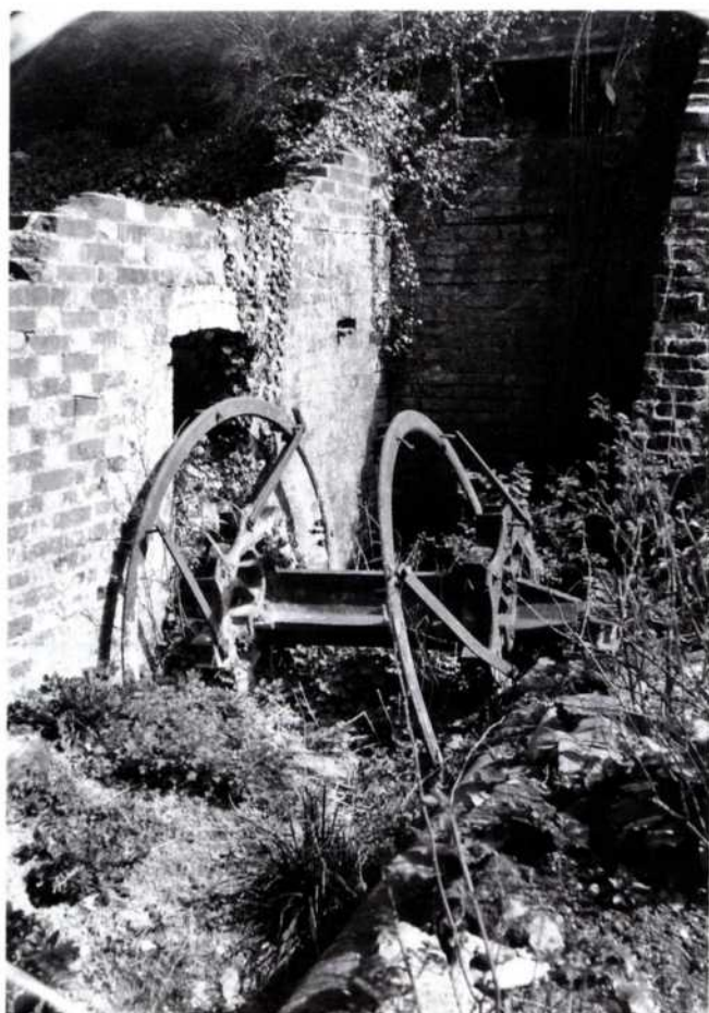
Fig. 1 Poynings Manor Mill, present condition of wheel and wheel pit
