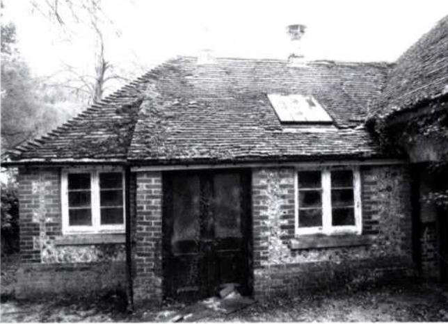
Fig. 1 The Pump House (north side of Area A on key plan)
