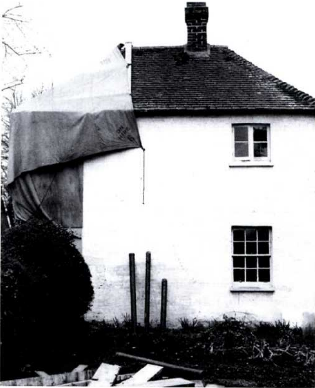
Fig. 9 Lyons Corner tollhouse, Slinfold, awaiting demolition April 1970
