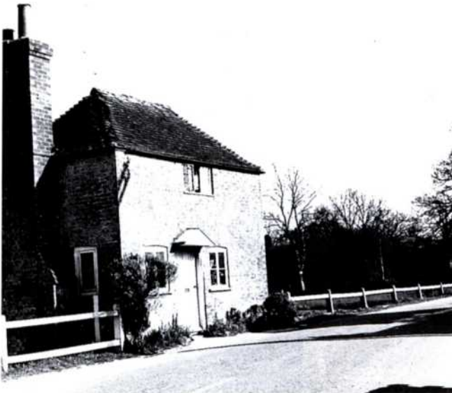
Fig. 4 Loxwood tollhouse March 1938
